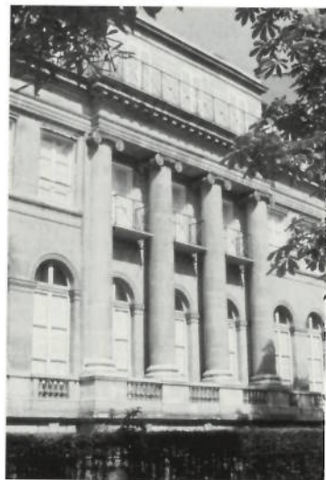
2.44. Town house, Avenue Gabriel, Paris, 1780. Lemoine de Couzon. Unobtrusive metal guardrails are appropriate on the three balconies added at the second story at a later date. Metal brackets also support the thin stone slabs.
