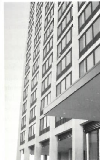
2.32. Apartment building, Num's Island, near Montreal, 1969. Mies van der Rohe. The section of the steel supports is reduced above the third regular story and again above the eighth story.
