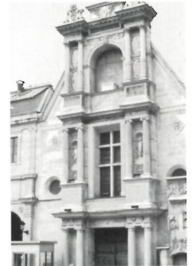
2.33. The central bay of the chateau at Anet, west of Paris, 1455–1555. Philibert Delorme. Re-erected at the Ecole des Beaux-Arts, Paris, 1804. An elegant sequence of superposed Doric, Ionic, and Corinthian twin columns. Although receding towards the wall, the axes of superposed columns remain in the same vertical plane perpendicular to the wall.
