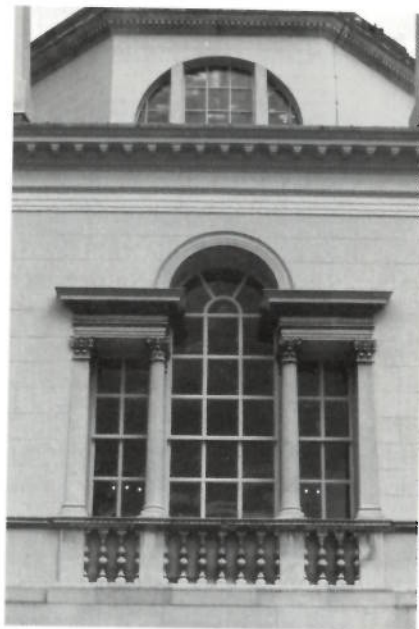
2.50. Chiswick House, near London, 1725–29. Lord Burlington with William Kent. Palladian window with a thermal window above in the drum.
