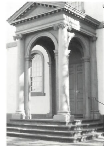
2.28. Touro Synagogue, Newport, Rhode Island, c. 1763. Peter Harrison. An Ionic porch showing the relationship of Ionic capitals and modillions. The modified Ionic capitals are of the "Scamozzi" type. Note how the rear columns are engaged in the back wall.
