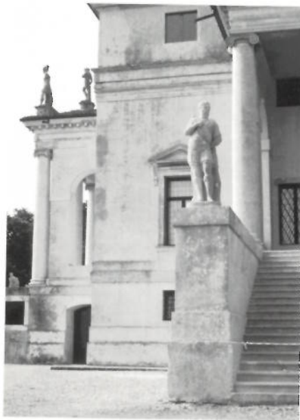
2.36. Villa Rotonda, near Vicenza, 1566. Andrea Palladio. One of eight simplified pedestals, each supporting a statue. What appears to be a pedestal stretches out to form the base of the entire building. The design of the attic story resembles that of a pedestal; it can be glimpsed above the entablature.
