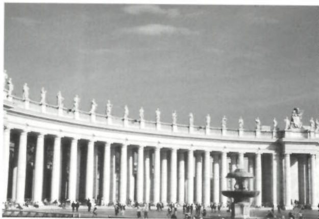
2.25. St. Peter's Square, Rome, begun 1656. Bernini used 280 columns, each 50 feet high, to unify a huge and complex urban space. The architect combined Doric columns with an Ionic entablature.
