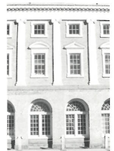
2.22. A pediment that is too large will overwhelm a building by its excessive mass.
