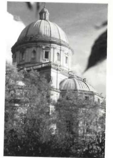
2.59. S. Maria della Consolazione, Todi, near Perugia, begun in 1509. Attributed to Bramante or Baldassarre Peruzzi. A remarkable essay in pure geometry, it consists of a cube surmounted by a cylinder capped by a half-sphere. Semi-domes are applied to all four lateral faces of the cube.
