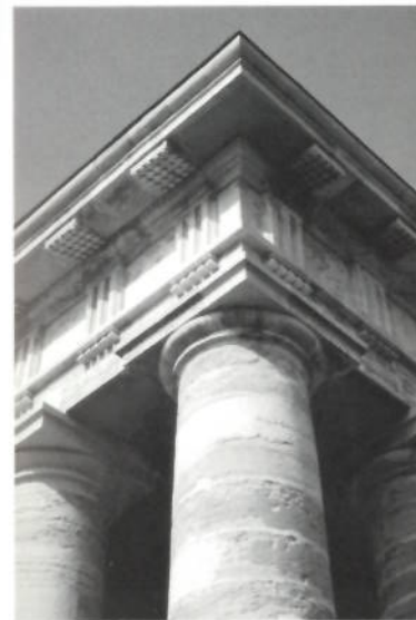
2.27. A corner of the entry building at the Royal Saltworks. In the Doric order, the spacing of columns is determined by mutules, triglyphs, and metopes or by dentiles.
