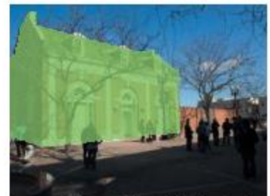
proposed site. existing building to be demolished.
